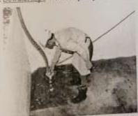
ge 3: High Pressure Washing. The ceilings and walls of the water tanks are cleaned using a high pressure washer.
