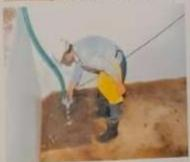
Stage 3: High Pressure Washing. The ceilings and walls of the water tanks are cleaned using a high pressure washer.
