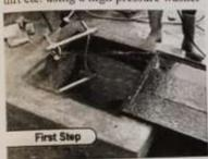
2: Dewatering. Water is pumped out of the tanks with hygenic method using an specially designed pump.
