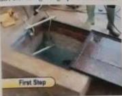
Stage 2 : Dematering. Water is pumped out of the tanks with hygenic method using an specially designed pump.
