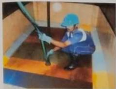
Sage 5: Vacuum Cleaning. The floor of the tank is cleaned using a high pressure washer and a wet vacuum cleaner.
